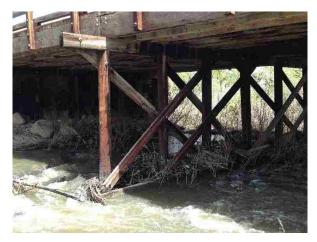
Figure 93. Street View of Bridge No. 1190 Showing Running Water Surrounding Intermediate Bent during the First Visit
