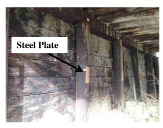
Figure 103. A Steel Plate Attached to Pile 10
